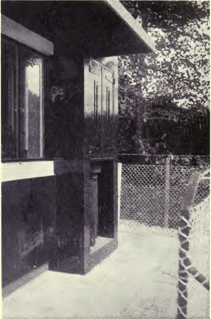
Foreign beat communication equipment: The Hague, Netherlands. Police booth, exterior view, showing how doors only cover upper section (about two-thirds the height of the entrance) so that the lower part remains open and may be inspected from the street.
